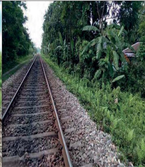
*Figure 2.14: NFR: Vegetation along the track in section RVK-APDJ section*
