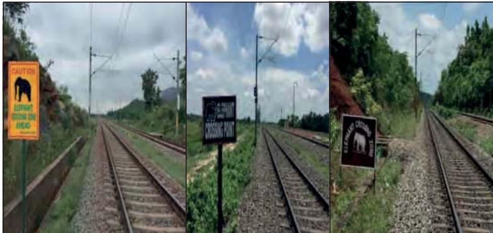
Figure 2.15: ECoR: Retro reflective signage board in Kendujhar Garh - Basantapur section
